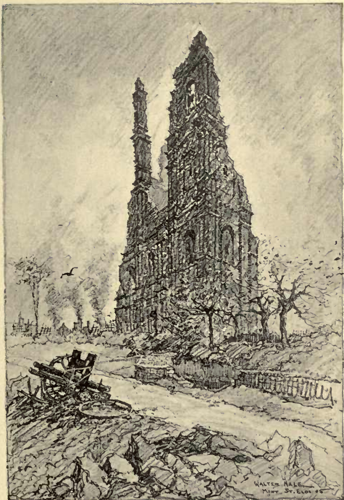
THE ROAD THROUGH MONT ST. ELOI.
